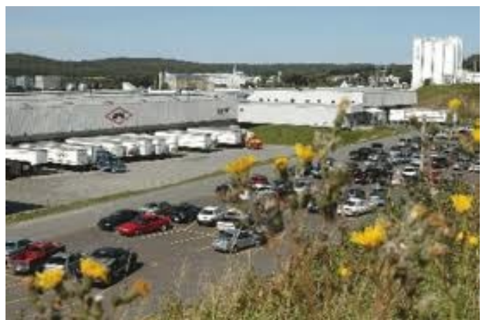
IPL Inc.—Operation plant of the Industries located at St. Damien-de-Bellechasse where they manufactured the plastic pieces. This is where Jean-Marie Chabot started his career as engineer in 1967 in the family business created by Émile Métivier.
